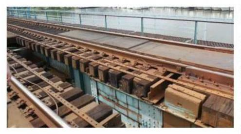
Metro-North began work in the spring of 2016 to replace the existing miter rails, the bridge timbers on all tracks and install the expansion rails.
